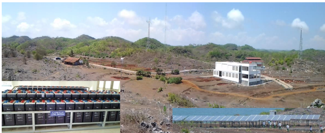
Fig. 6: Baron Technopark, wind-PV-Diesel (Source: Soeripno)
