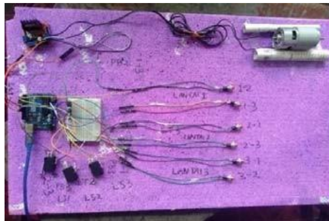
FIGURE 3. Three-Story Elevator Control System Design Installation
