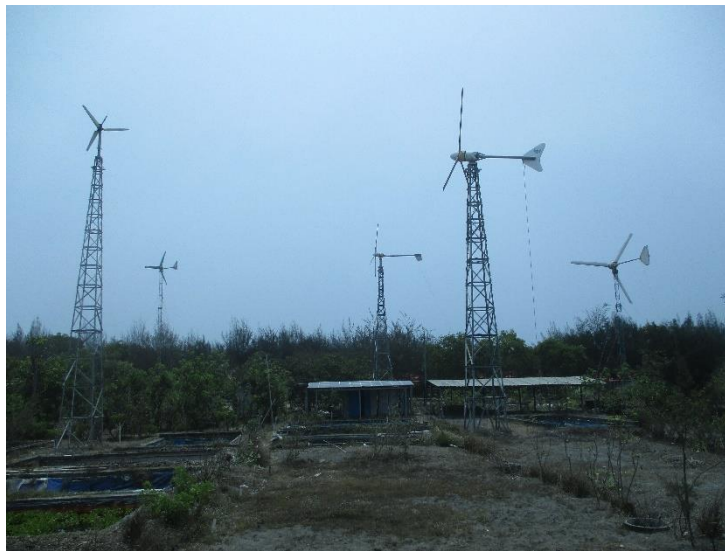
Fig. 7: Pantai Baru hybrid system of Wind-PV-Diesel for ice making (Source: Soeripno)
