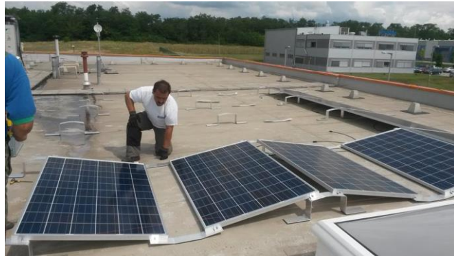
Fig. 10.b. Flat fixation of PV module installation, NVS (2014)
